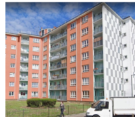
Southwark Park Estate
