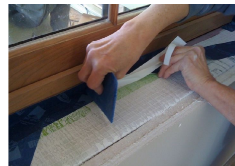
Air tightness . An important but still undervalued aspect of window installation
