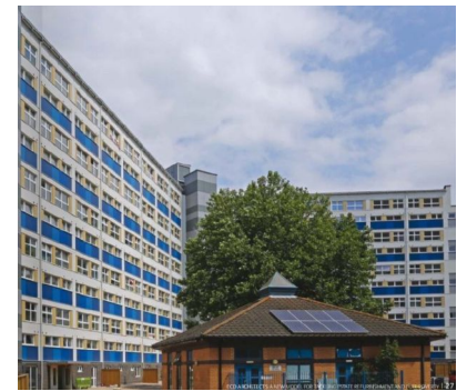
Wilmcote House, Plymouth City Council
