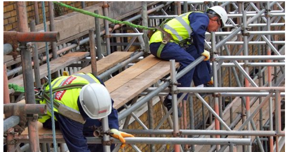
Scaffolding is a large part of the cost for replacing glazing. By including window upgrades as part of routine maintenance and upgrade work, costs can be minimized.
