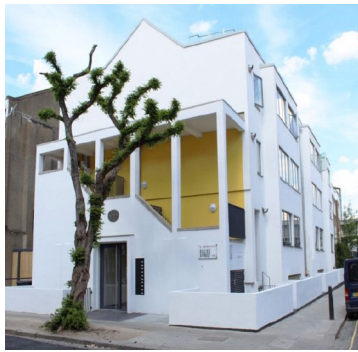
Artic Street, Housing Coop, Camden
