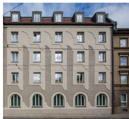
Munich. Housing block renovation.
